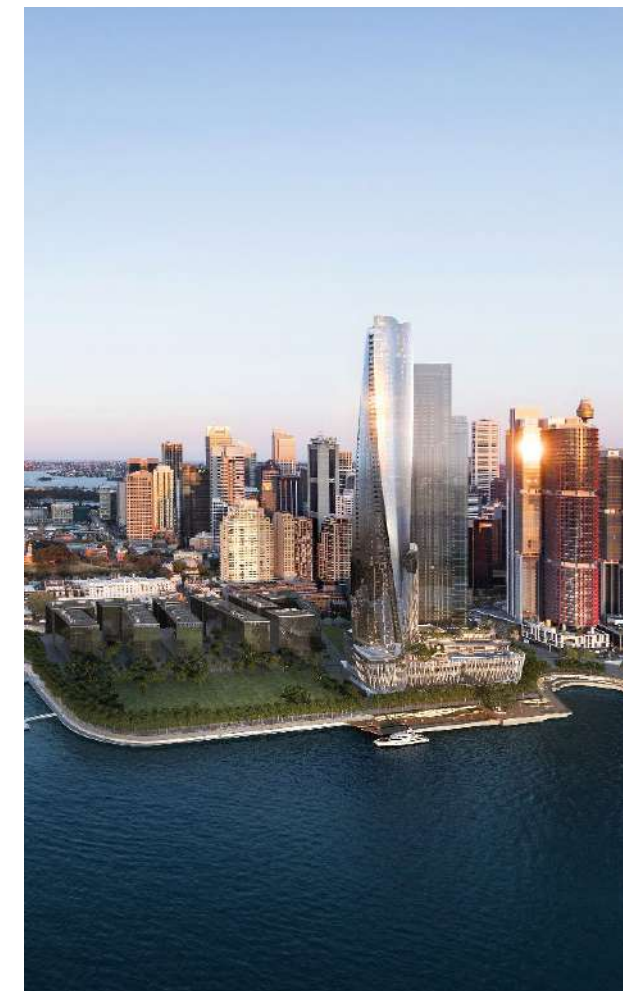
Large areas of public space have been created as part of One Barangaroo
